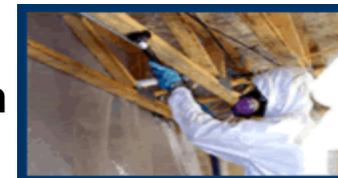
**Step1: Inspection** to determine source and severity of problem. Includes air, swab and tape lift sampling, borescope and visual inspection, moisture mapping, thermal imaging, relative humidity check and building analysis.
