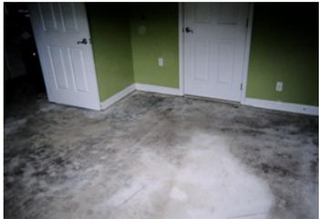
Indoor Air Quality Testing indicated elevated levels of mold. Further investigation uncovered potentially toxigenic mold under a hardwood floor growing on the sub-floor.
