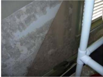
Indoor Air Quality Testing indicated elevated levels of mold and further investigation uncovered potentially toxigenic mold behind wall paper.
