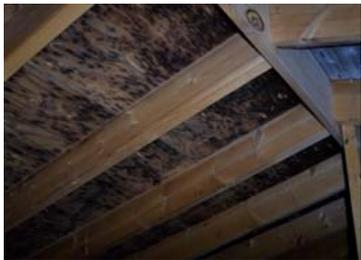
Indoor Air Quality Testing indicated elevated levels of mold and in the home the tape lifts verified hypoallergenic mold in the attic growing on the sheathing.
